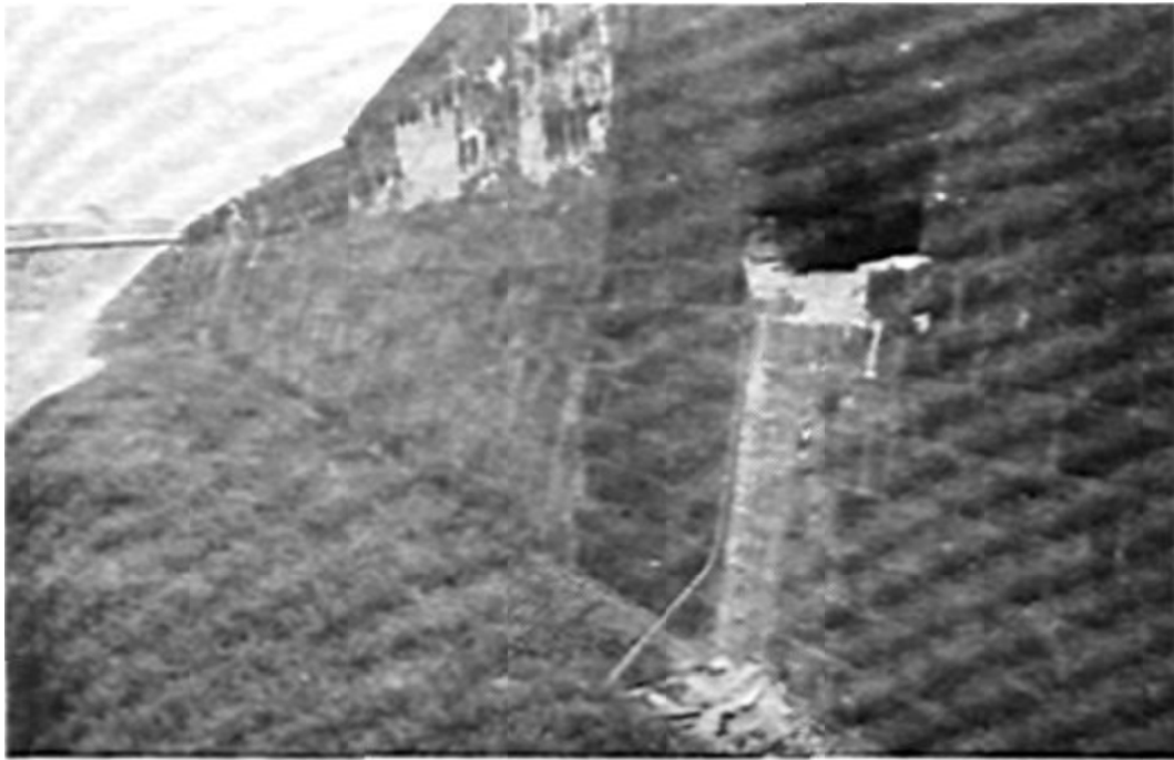
Typical section of wall of Intramuros, showing firing slit, 40 feet thick at the base, tunnelled walls were excellent for defense. (Field Artillery Journal photo)
