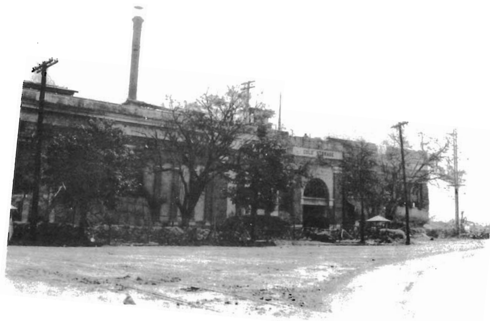
Ice Plant Building Annex 7
