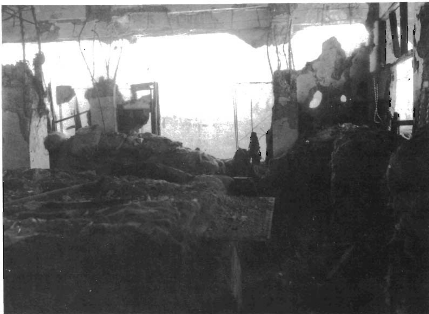
Room in Santa Teresa College Annex 14
