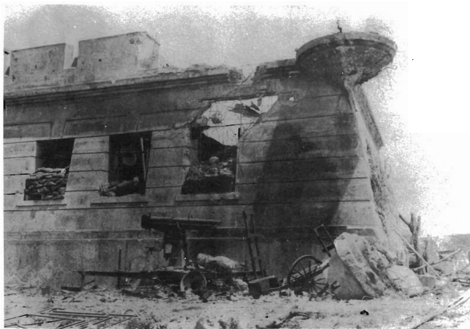
S7 corner of New Police Station Annex 16
