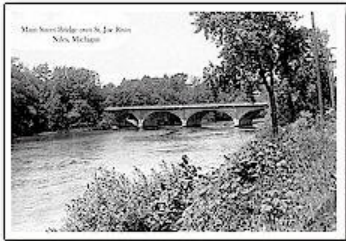
Main St. Bridge over St. Joe River Niles, Mich.
