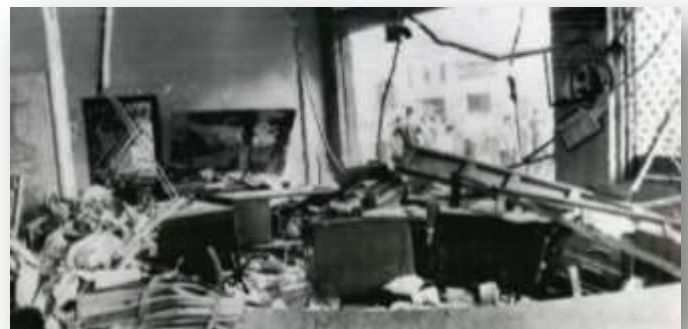
March 30, 1965. Wrecked interior of Embassy in Saigon.
