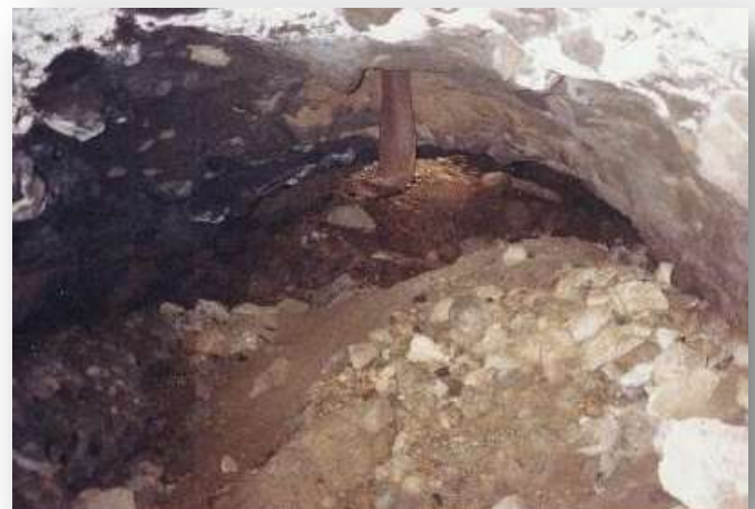
Diesel exhaust vent
