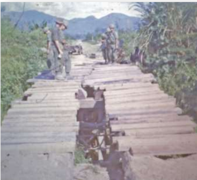
Aussie Engineers repair bridge at Than Duc
