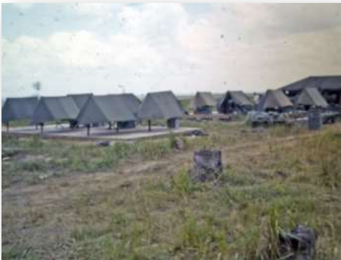
Construction of Camp Zinn underway.
