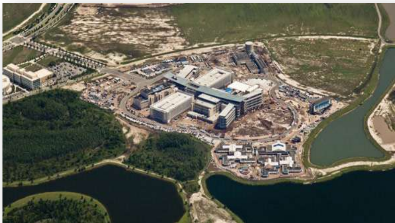
New Orlando area VA hospital under construction
