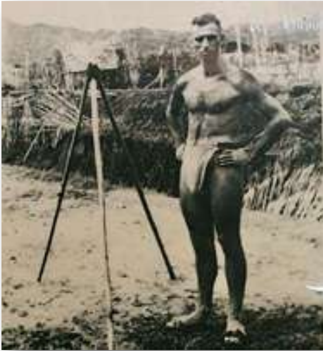
An allied P.O.W. wearing only loin cloth stands alongside primitive tripod used for leveling ground for the Thai-Burmese railway.
