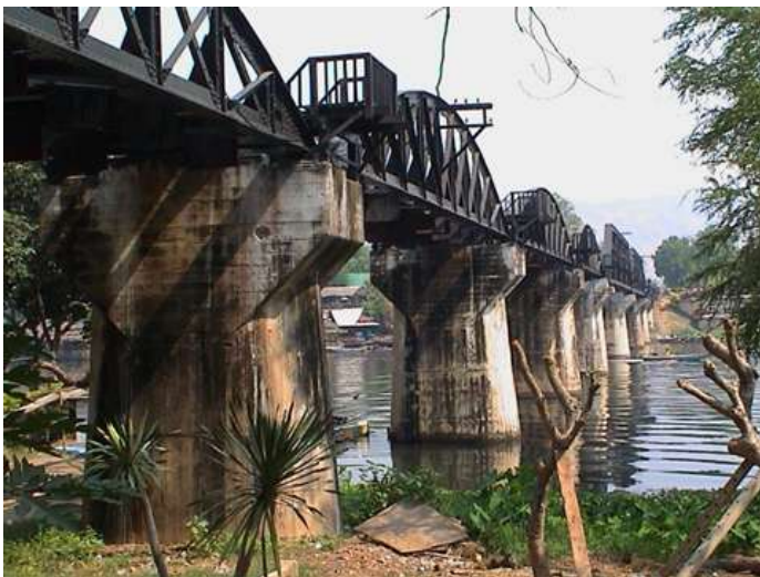
The bridge over the River Kwai in June 2004. The round truss spans are the originals; the angular replacements were supplied by the Japanese as war reparations.
